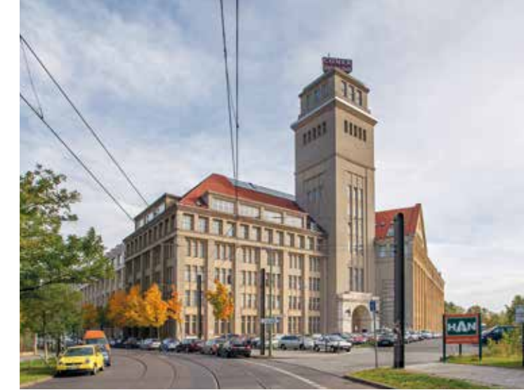
Comer Business Park, Peter-Behrens-Bau
